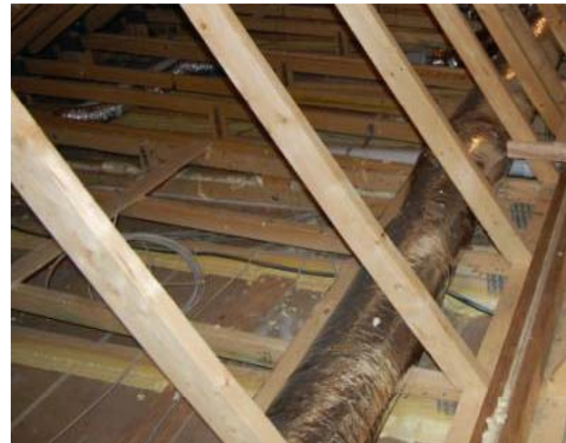
■ After ceiling drywall
