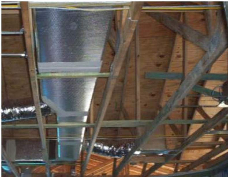
■ Before ceiling drywall
